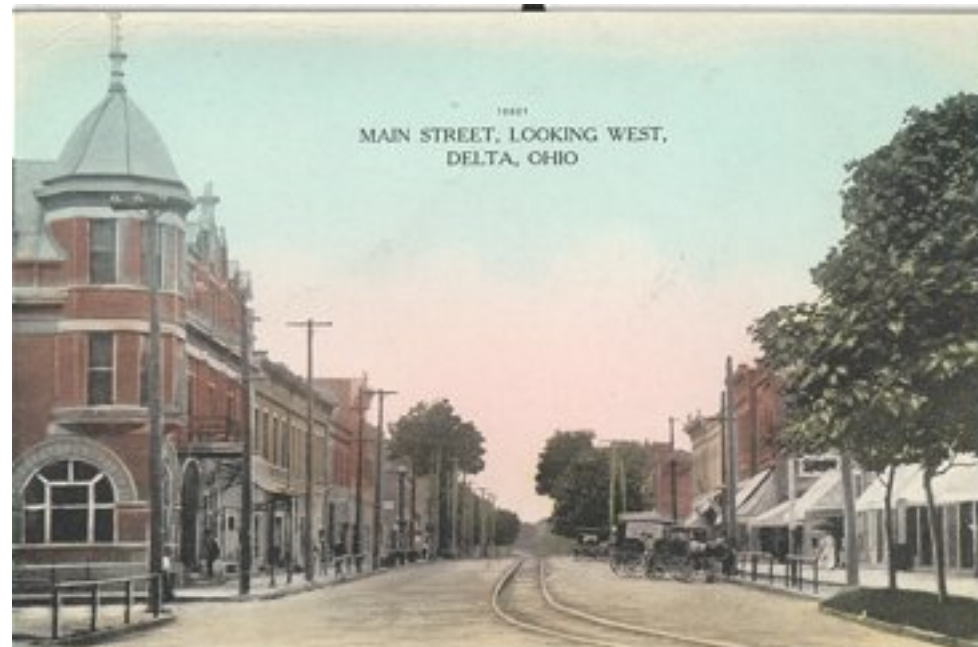
Looking West on Main Street of Delta
